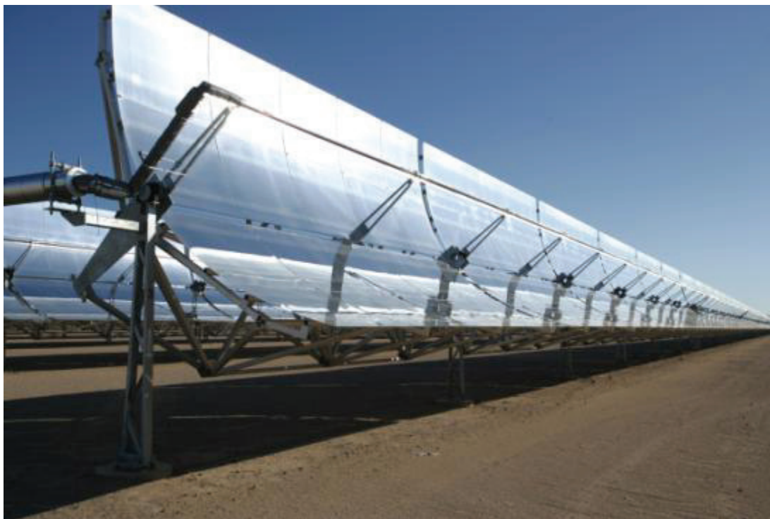
FIGURE 5.10 A parabolic trough concentrator solar thermal plant in Nevada. SOURCE: Courtesy of Acciona Solar Power.
