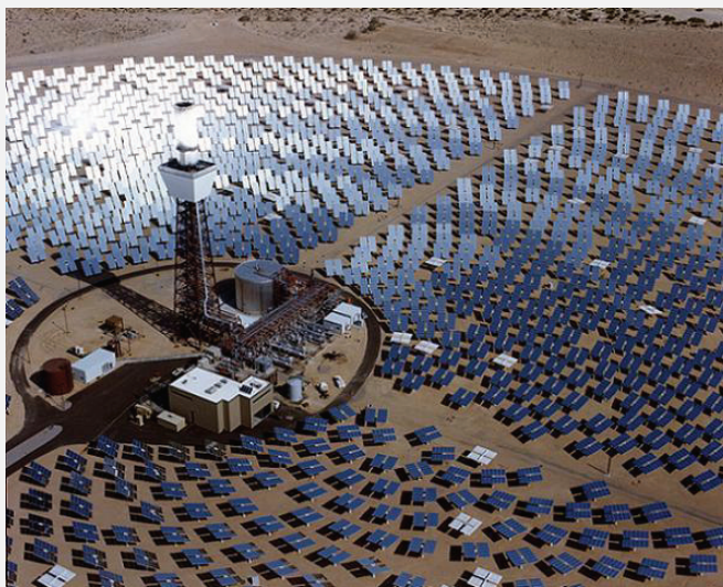
FIGURE 5.2.1 In this photograph of a concentrated solar power (CSP) technology, stretched membrane heliostats with silvered polymer reflectors will be used as demonstration units at the Solar Two central receiver. The Solar Two project will refurbish this 10-megawatt central receiver power tower, known as Solar One. SOURCE: Image available at https://www.eeremultimedia.energy.gov/solar/ . Accessed June 5, 2012.
