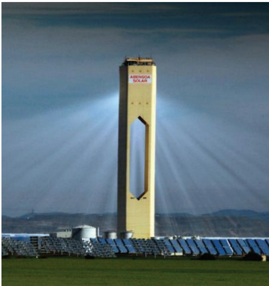
FIGURE 5.11 11 MW Solar Power Tower near Seville, Spain. SOURCE: Courtesy of Abengoa Solar.
