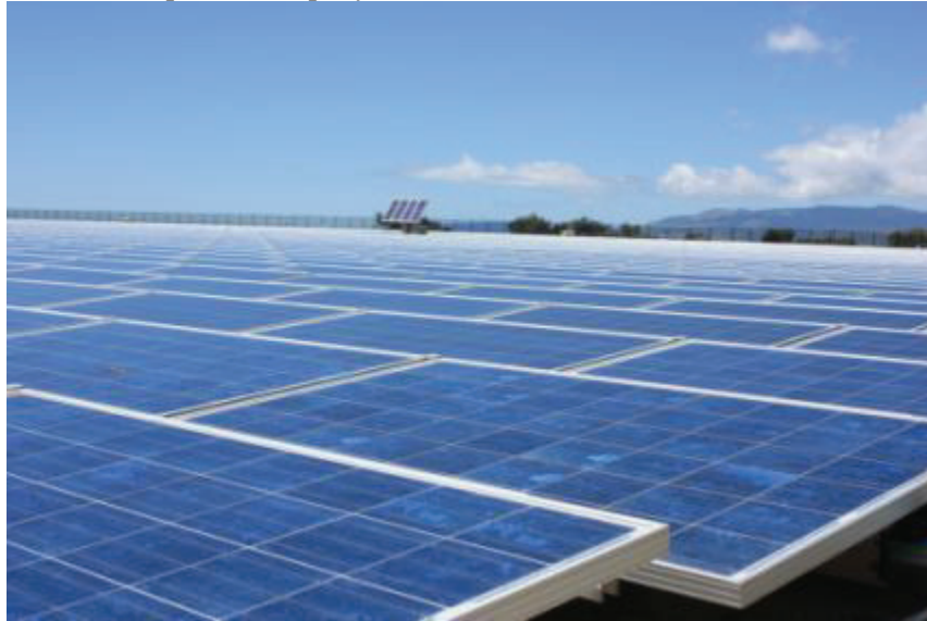
FIGURE 5.5 Silicon solar cells deployed for utility power production. SOURCE: Courtesy of Suntech Power Holdings, Inc.
